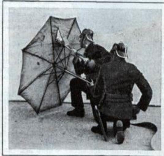
This large type of asbestos umbrella permits several hose nozzles to be thrust through it, protecting firemen from heat.
